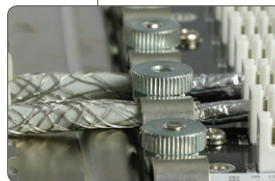
Raised metal tray improves better contact resistance and transfer impedance.
